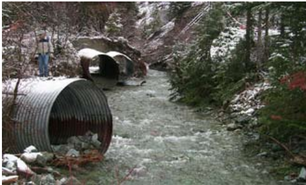
The choice is clear: culvert blowouts (left) or careful road decommissioning (right). U.S. Forest Service photos
