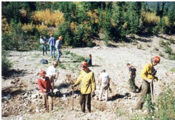
Workers hand-plant native vegetation on a decommissioned road on the Flathead. Keith Hammer photo
