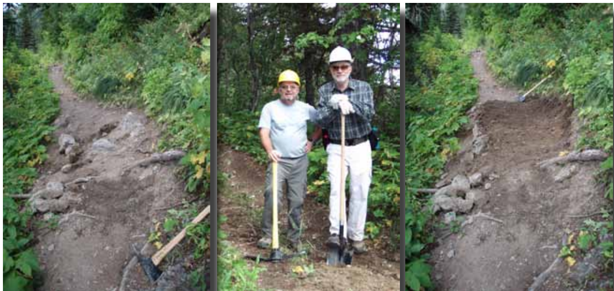
A couple Swan Rangers do volunteer trail repair on the Peters Ridge Trail (center). Before (l) and after (r) photos of repairs made to the Strawberry Lake Trail! Keith Hammer Photos
