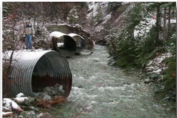
Road reclamation carefully removes culverts (left), rather than letting them blow out. Forest Service photos
