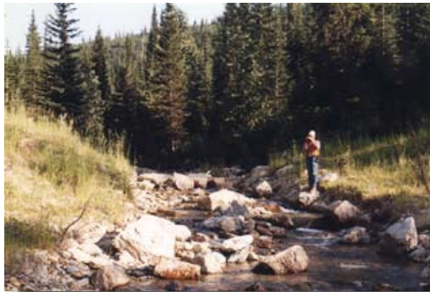
Road reclamation carefully removes culverts (left), rather than letting them blow out. Forest Service photos
